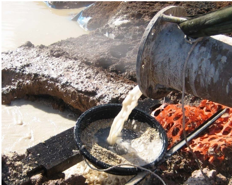
Figure 4.4: Drilling fluid and drill cuttings exiting the mud system (PEL433 Allambi-1C)
