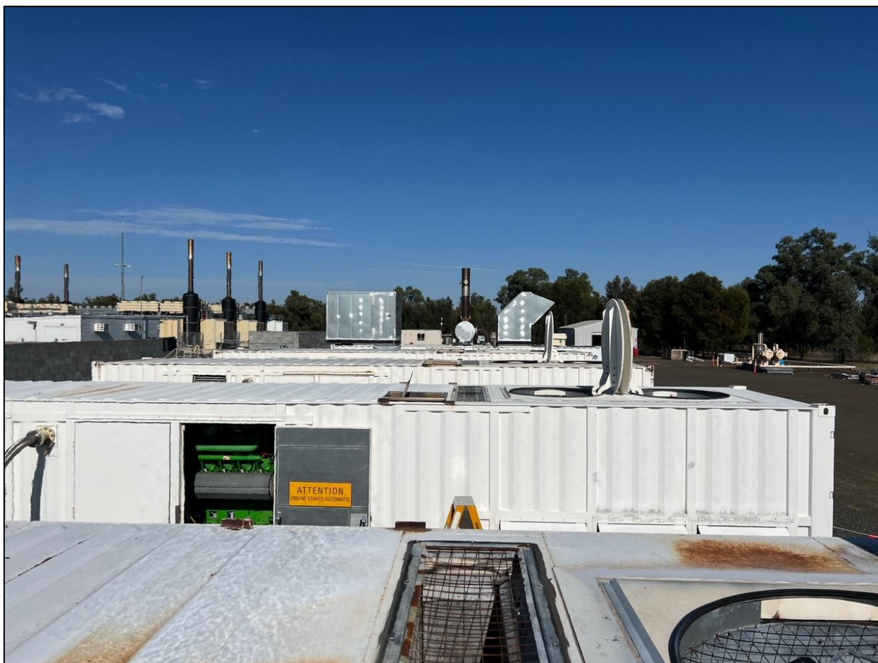
Figure 2: IMW Generator Stack Release Points
