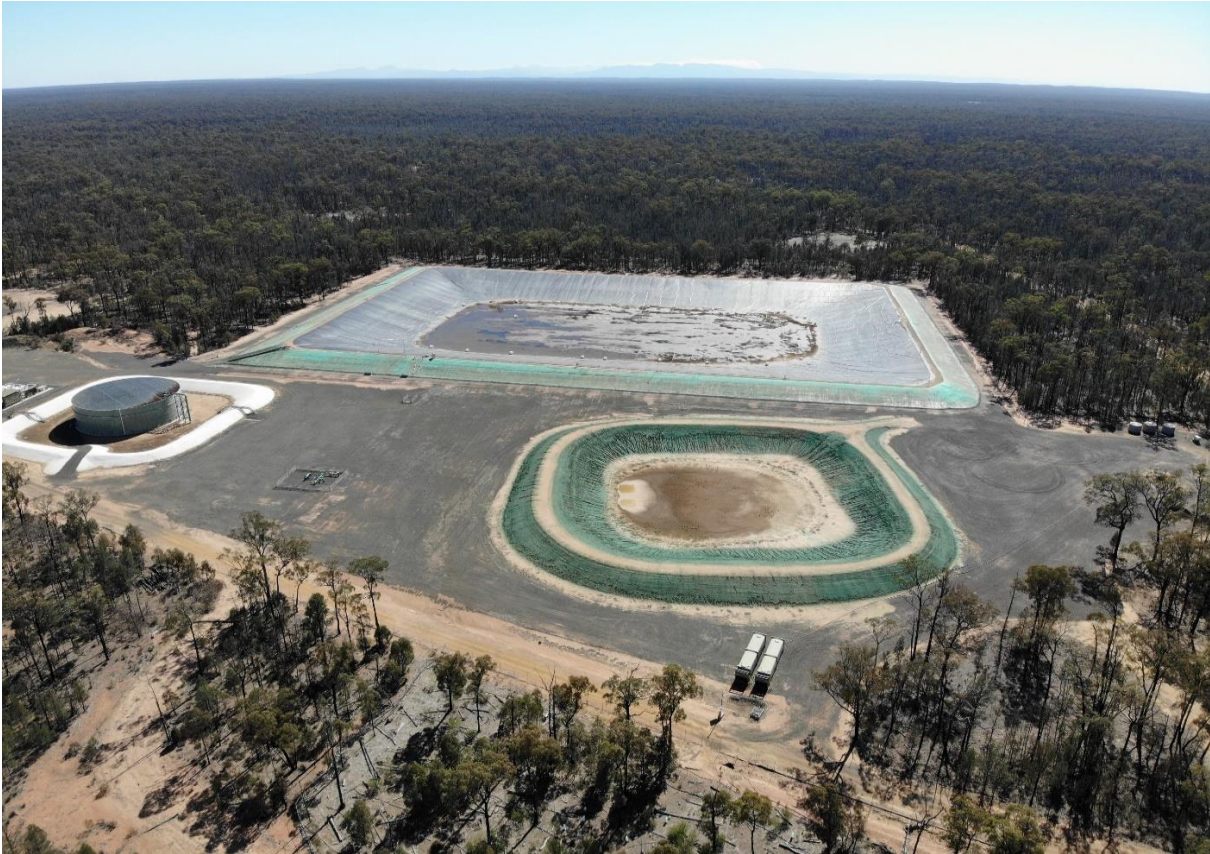
Figure 6.1 - Aerial view of infrastructure at Bibblewindi
