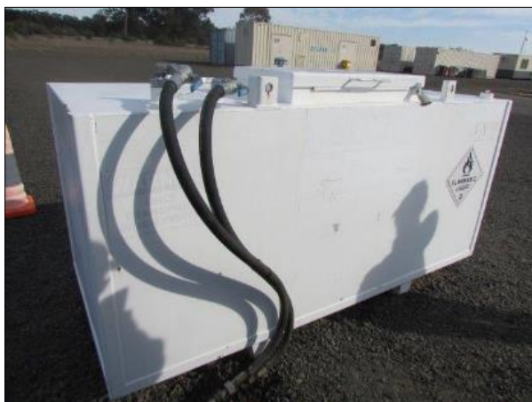
Photo 29 – Self-bunded bulk fuel storage facility at the Leewood Facility RO Plant (22 August 2023)
