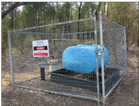
Photo 19 – Low point drain container Dewhurst 27 (22 August 2023)
