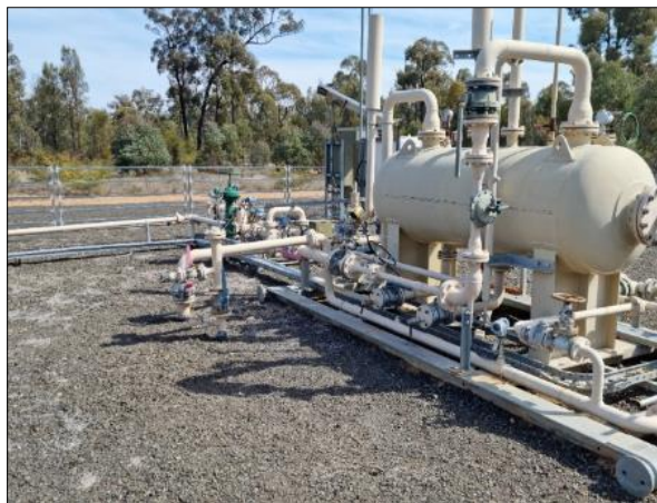
Photo 41 – Dewhurst 16 gas gathering equipment and meters (22 August 2023)
