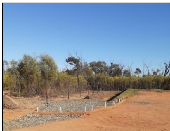
Photo 14 – Dewhurst 43 Well Pad ESCP additional controls (25 August 2023)
