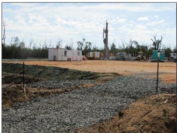
Photo 13 – Dewhurst 43 new well pad and bunding (constructed) (22 August 2023)
