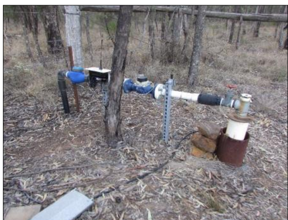
Photo 21 – Bibblewindi 5 groundwater bore and meters (22 August 2023)
