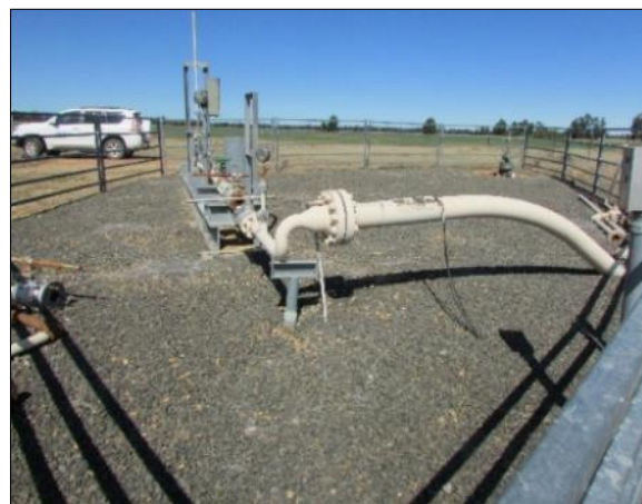
Photo 36 – Coonarah 4 Well Pad – Partial removal of well head gathering equipment (23 August 2023)
