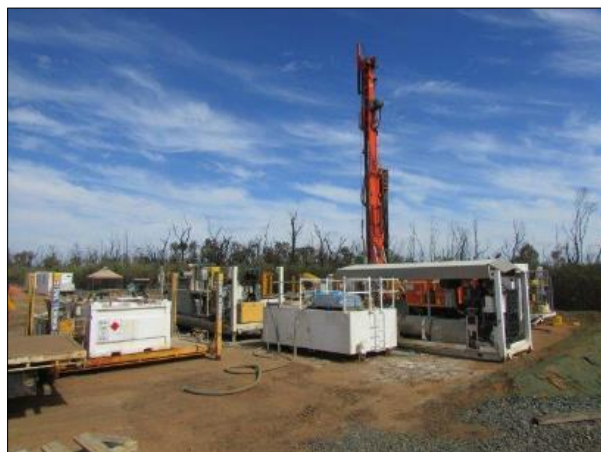
Photo 5 – Drilling of a groundwater monitoring bore at Dewhurst 43 (AECOM/Impax Drilling Services) (22 August 2023)
