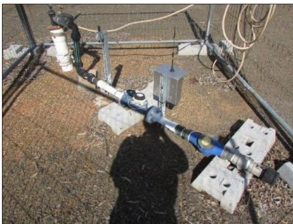
Photo 6 – Water extraction bore fitted with loggers/satellite telemetry for Santos and NSW Water (22 August 2023)
