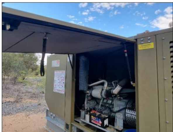
Photo 11 – Noise attenuated generator at Bibblewindi 5 (22 August 2023)
