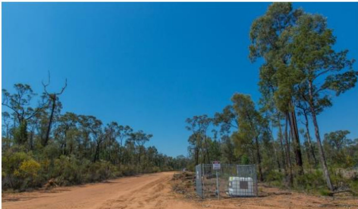
Figure 5.1 - Low point drain along gathering lines
