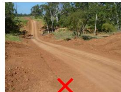
THIS WILL ERODE WHENEVER THERE IS GULLY FLOW, RESULTING IN ONGOING MAINTENANCE COSTS. IN ADDITION, THE SIDES OF THE TRACK WILL SCOUR DUE TO THE LACK OF STABLE DRAINAGE.
