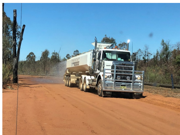
Photo 30: Tighes Gully Road, Piliga State Forest - Active dust mitigation around construction area of southern gas flow line construction
