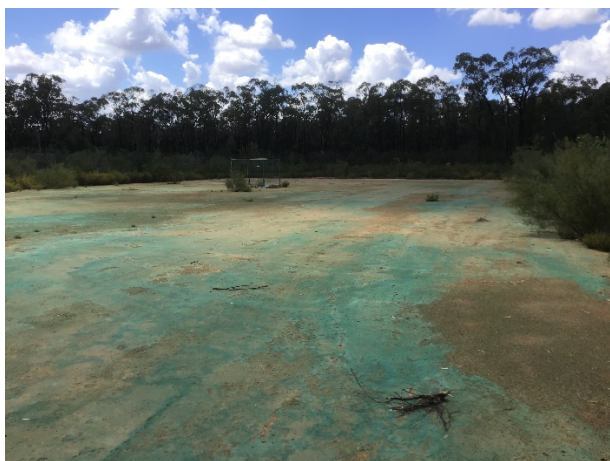
Photo 27: Dewhurst 31 – Cleared pad with cellar installed
