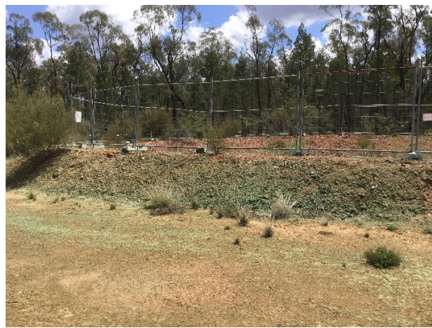
Photo 26: Dewhurst 30 – drilling mud storage (hasn't been used)
