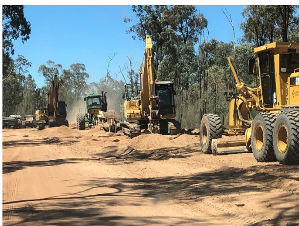
Photo 29: Tighes Gully Road, Piliga State Forest - Construction of southern gas flow line
