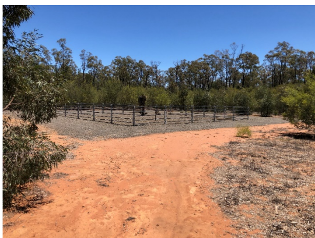
Photo 11: Dewhurst 13 – disused well head and pad
