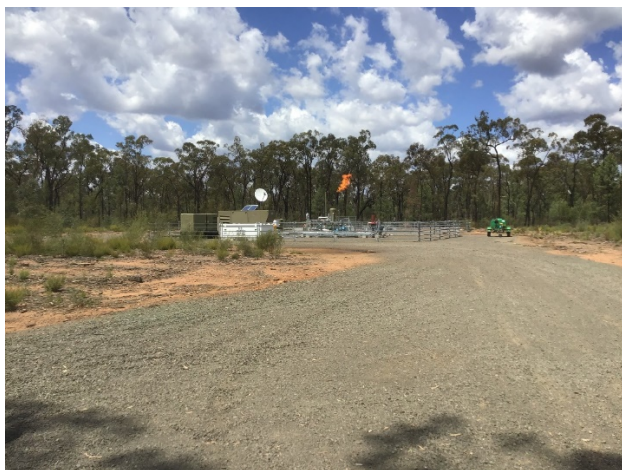
Photo 19: Dewhurst 28 – Well head, flare and facilities
