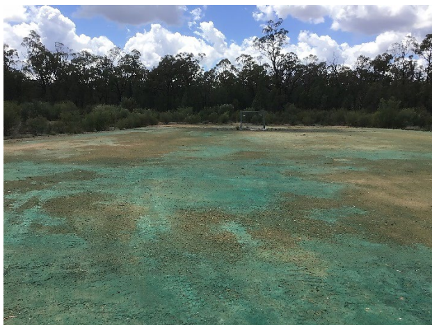
Photo 25: Dewhurst 30 – Cleared pad with cellar installed
