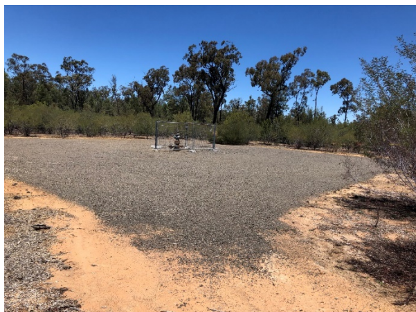
Photo 1: Dewhurst 18H - disused well head and pad
