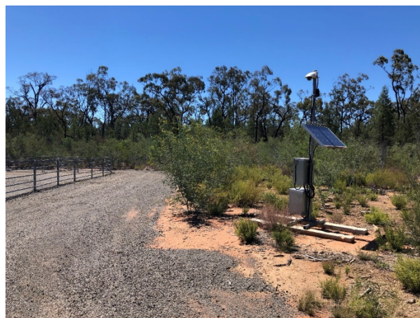
Photo 18: Dewhurst 27 – Rehabilitation, telemetry and CCTV
