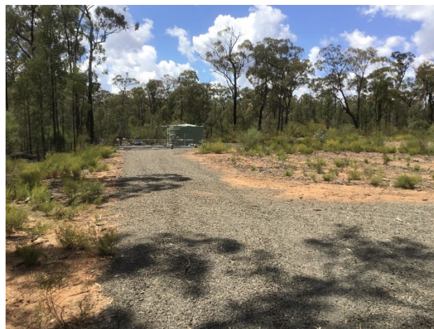
Photo 20: Dewhurst 28 - 22,000 L produced water balance tank
