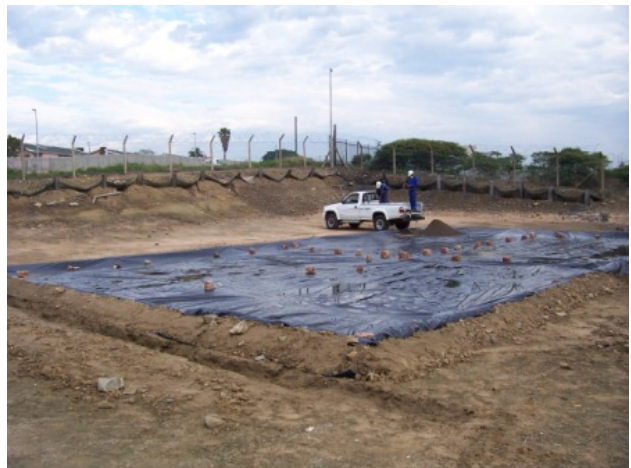
Plate 8. Landfarm during construction with impermeable (plastic) liner being applied
