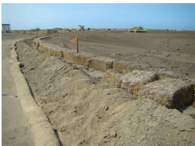
Plate 1. Earthen berm
