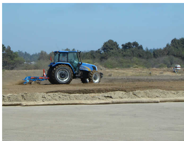
Plate 2. Tilling using a tractor attachment
