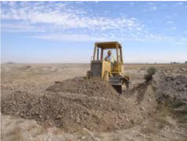
Plate 5. Dozer preparing landfarm site by moving topsoil and compacting the base
