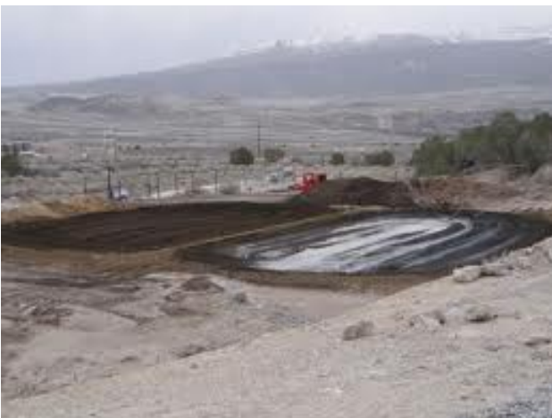
Plate 7. Two-cell landfarm - right hand landfarm has had recent application of heavily contaminated soil
