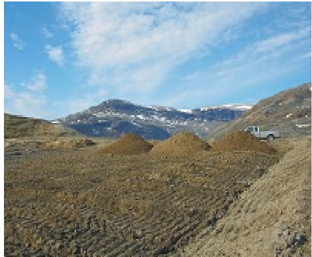
Plate 6. Active landfarm with stockpiled soil waiting for treatment at the rear and aerated, tilled soils in foreground
