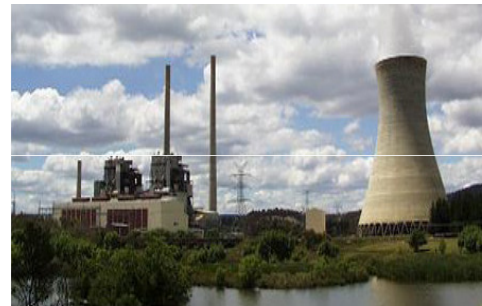
Wallerawang power station, NSW
