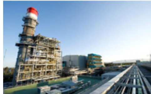
Tallawarra power station, NSW
