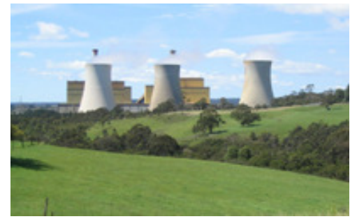
Yallourn power station, VIC
