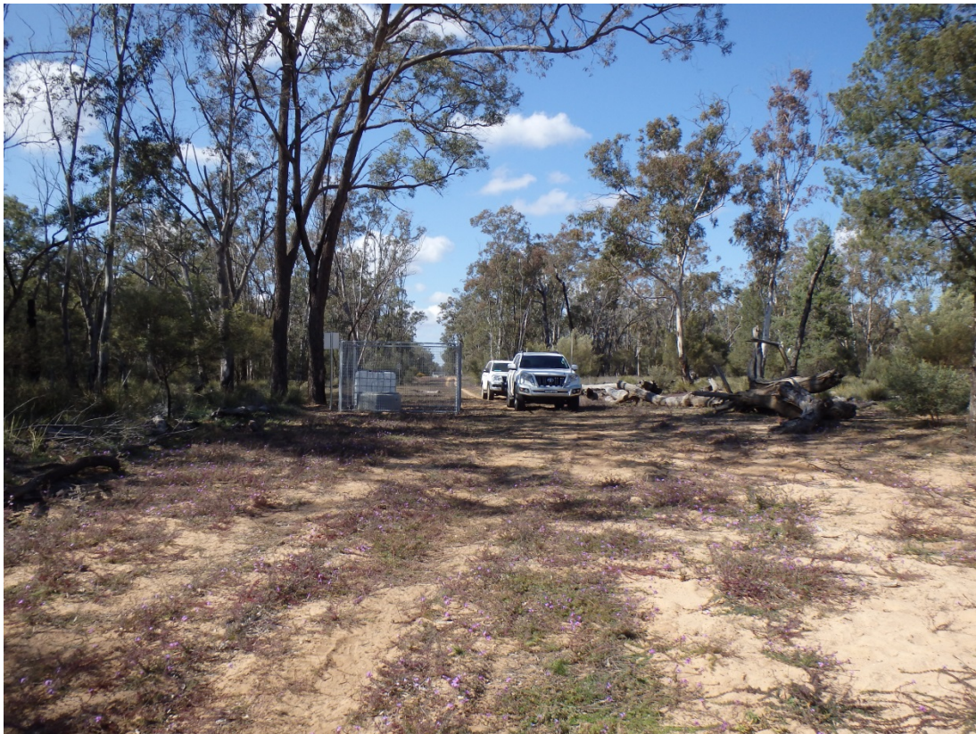
Plate 6 – Flow line route heading from Bohena Creek to Bibblewindi – note the fenced area containing a riser vent along the flow line
