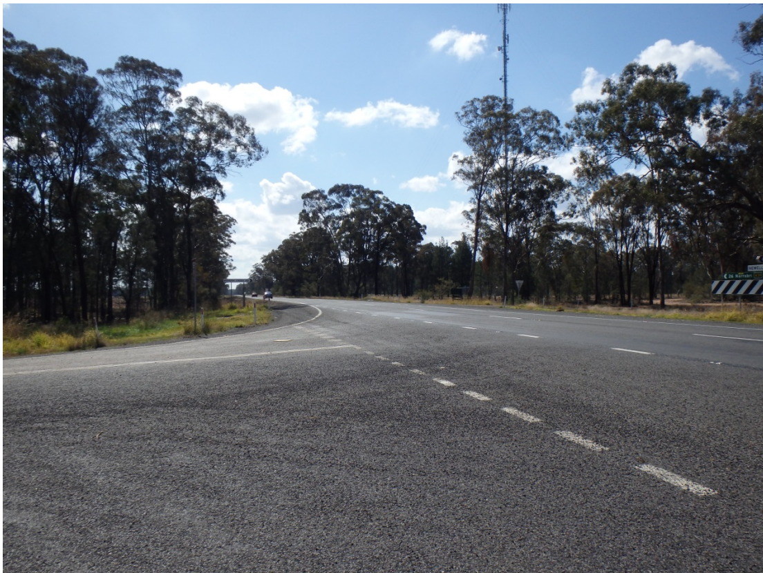
Plate 8 – Newell Highway/Old Mill Road intersection upgrade
