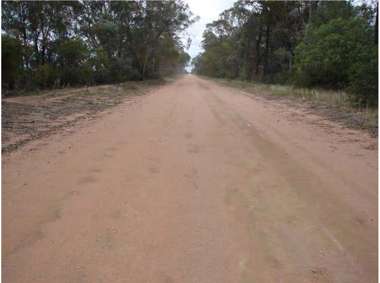
Photo 36 Nuable Road Facing West
