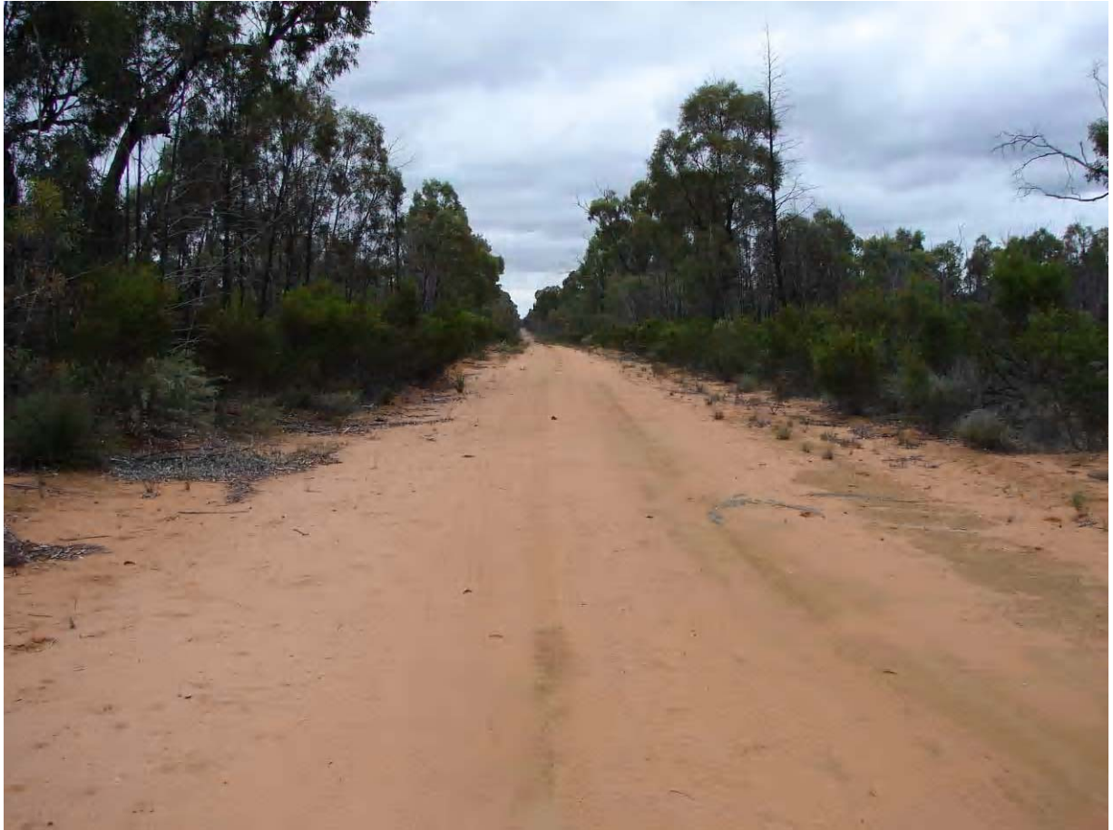
Photo 62 Worombi Road Facing North
