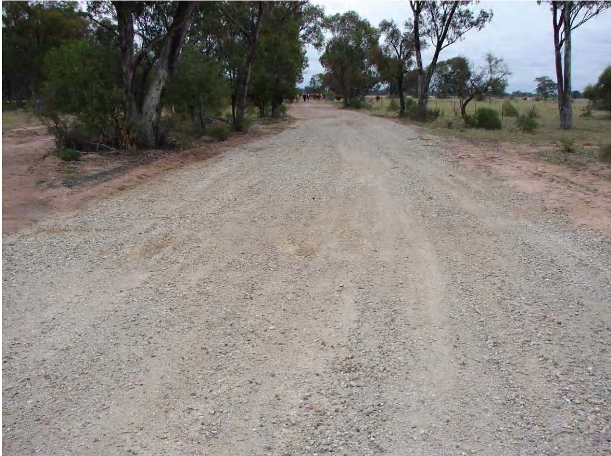
Photo 91 Power Station Entrance Road Facing West
