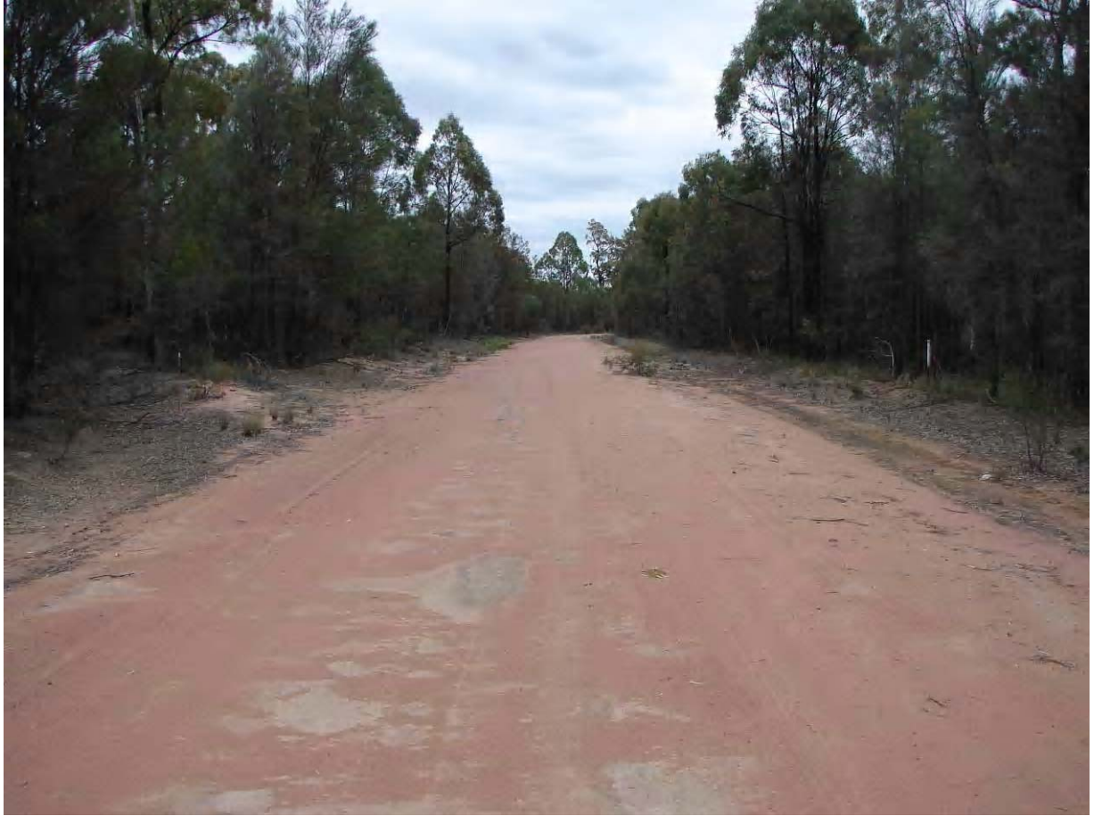
Photo 57 Apple Road Facing East at Pipeline Crossing
