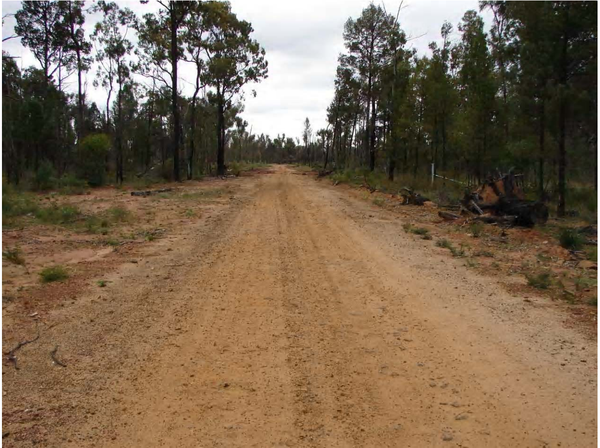
Photo 71 Gravel Road from Bibblewindi #2 Facing South
