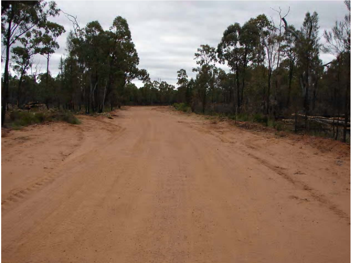
Photo 73 Garlands Road Facing South West
