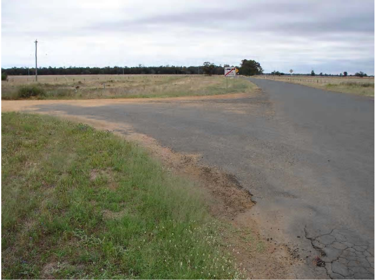
Photo 12 Kiandool Lane Intersection Facing West
