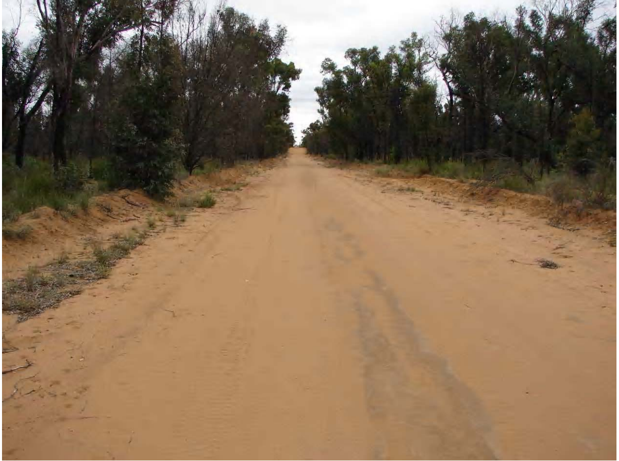
Photo 76 Middle Road Facing West
