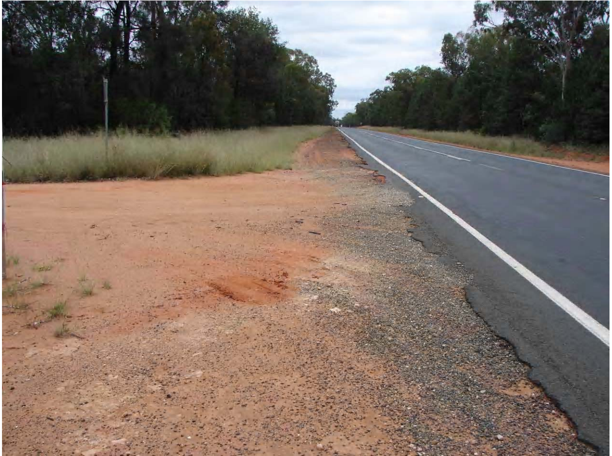
Photo 42 Glenwood Lane / Newell Highway Intersection Facing North
