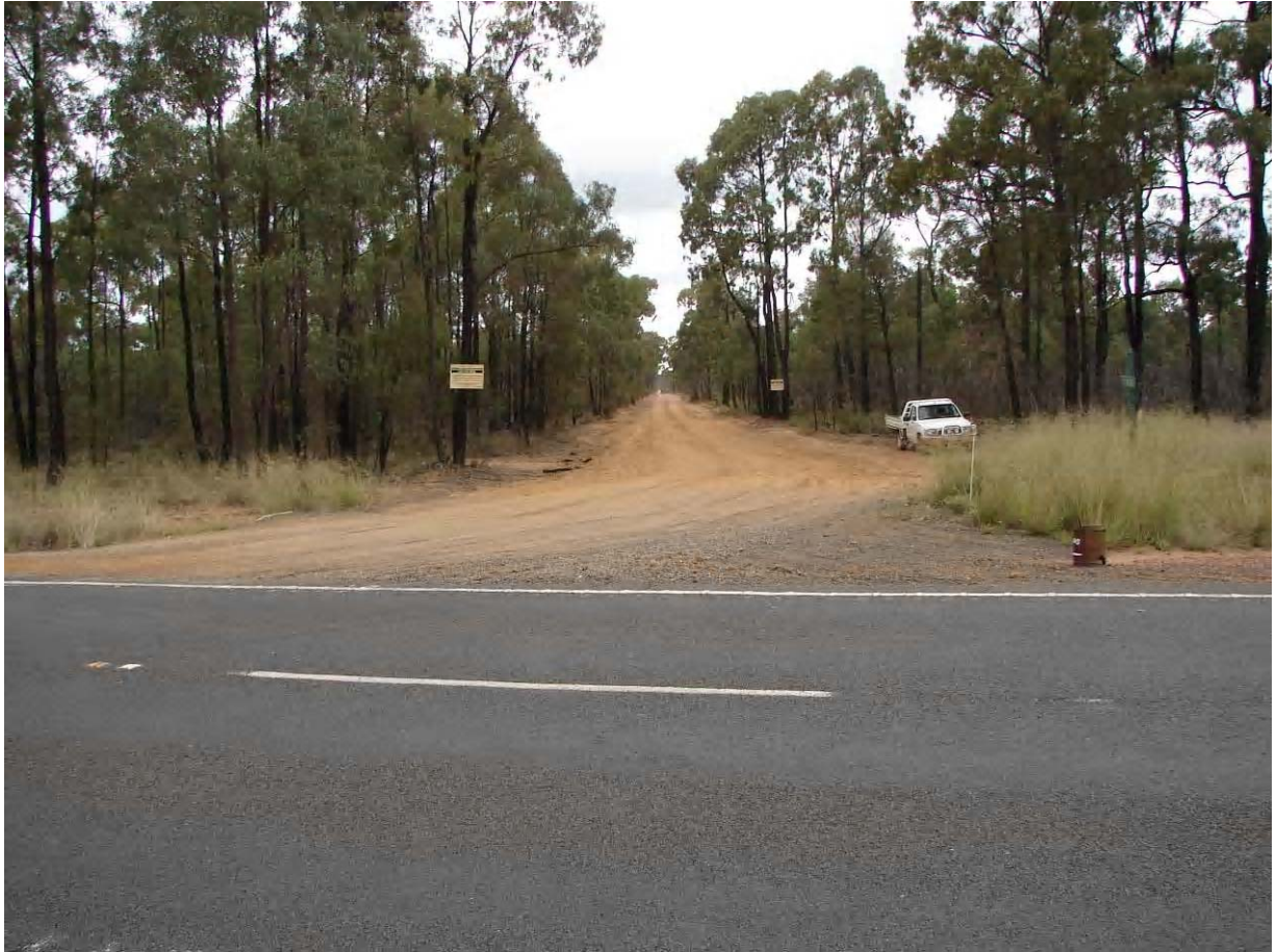
Photo 85 X-Line Road / Newell Highway Intersection Facing East
