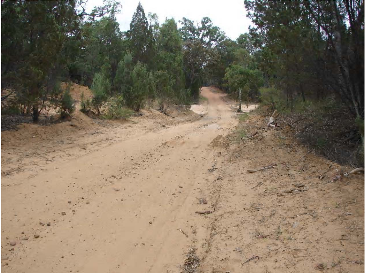
Photo 77 Creek Crossing on Middle Road Facing West
