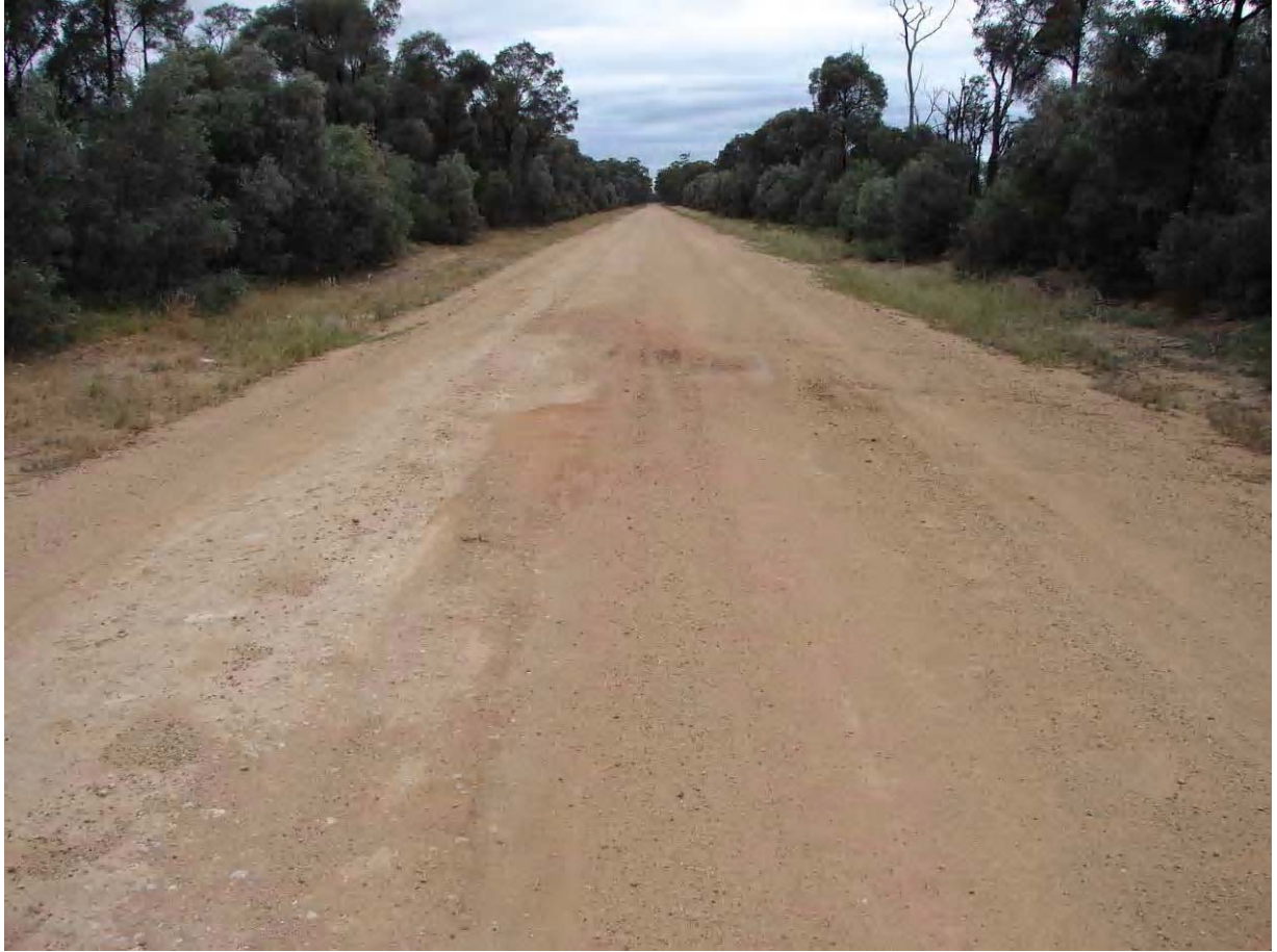
Photo 34 Nuable Road Facing East
