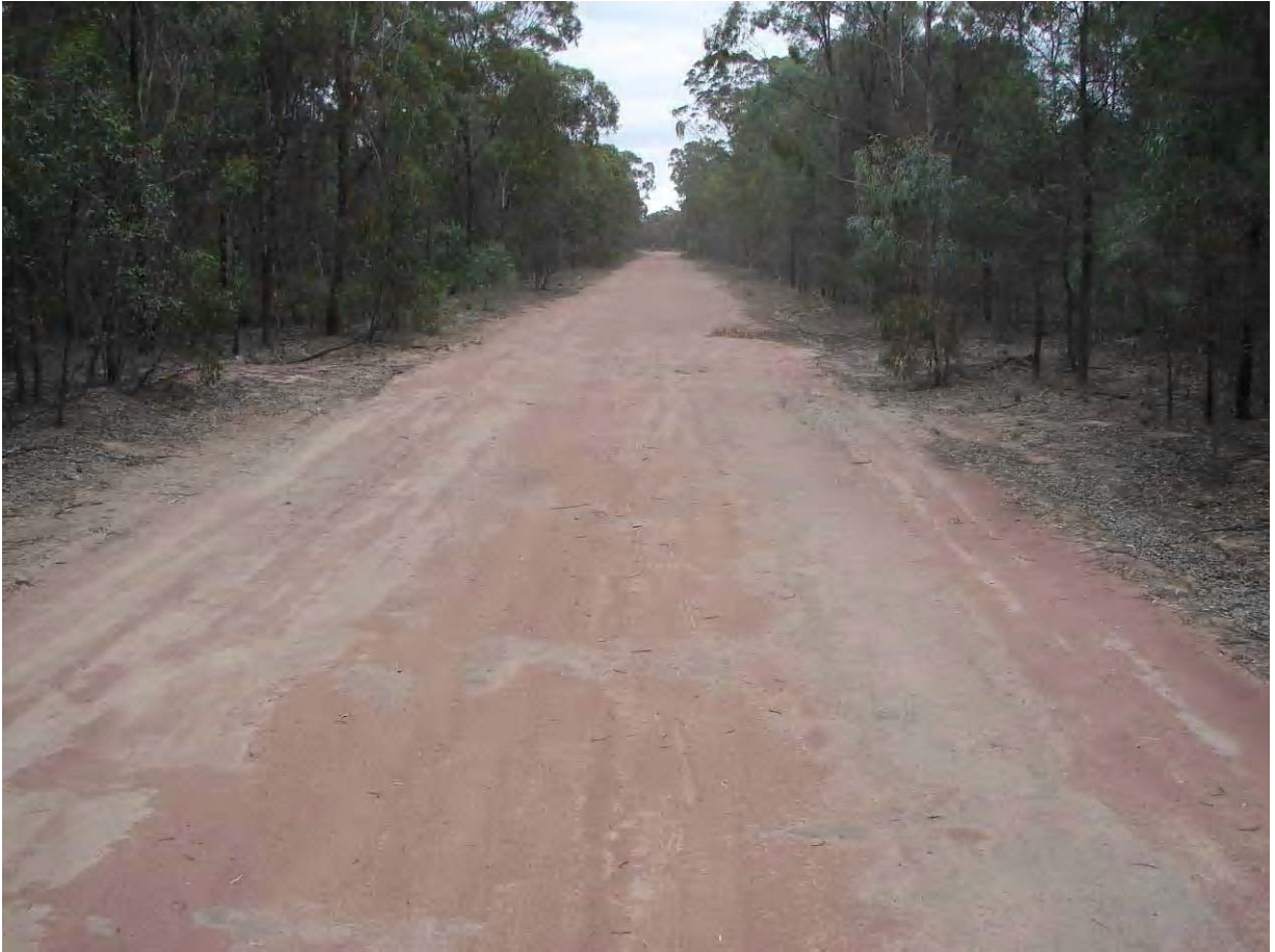
Photo 60 Worombi Road Facing North
