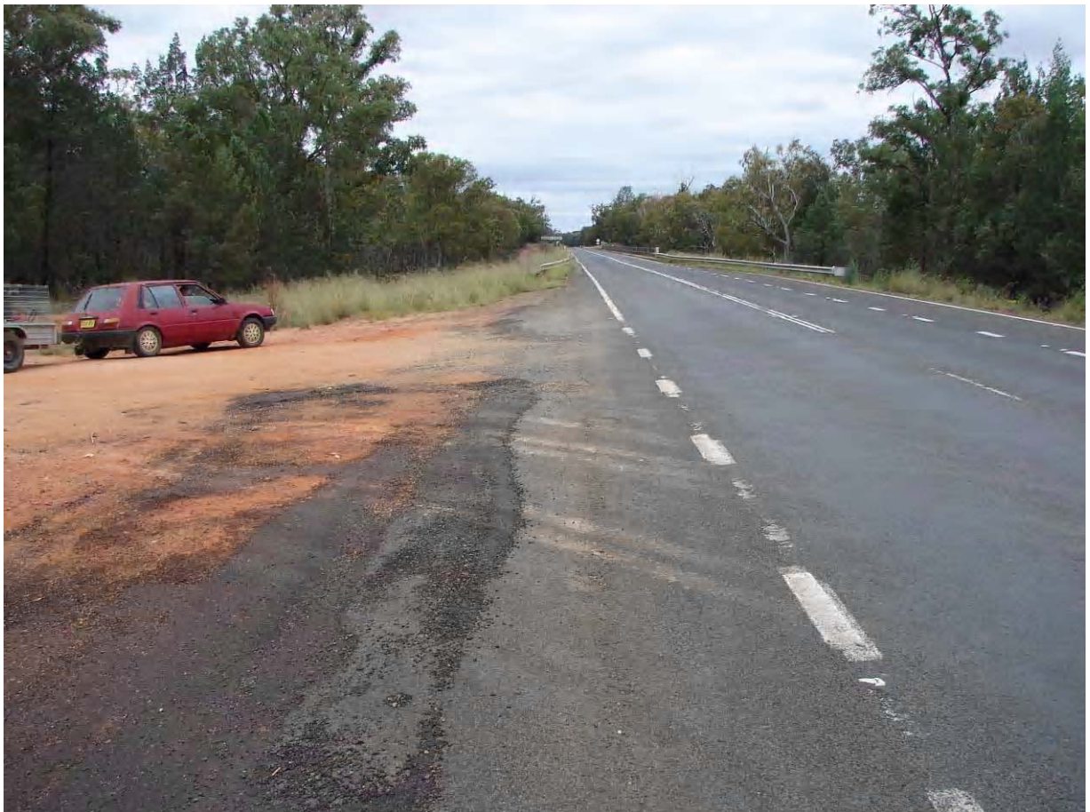
Photo 41 Cains Crossing Road / Newell Highway Intersection Facing North
