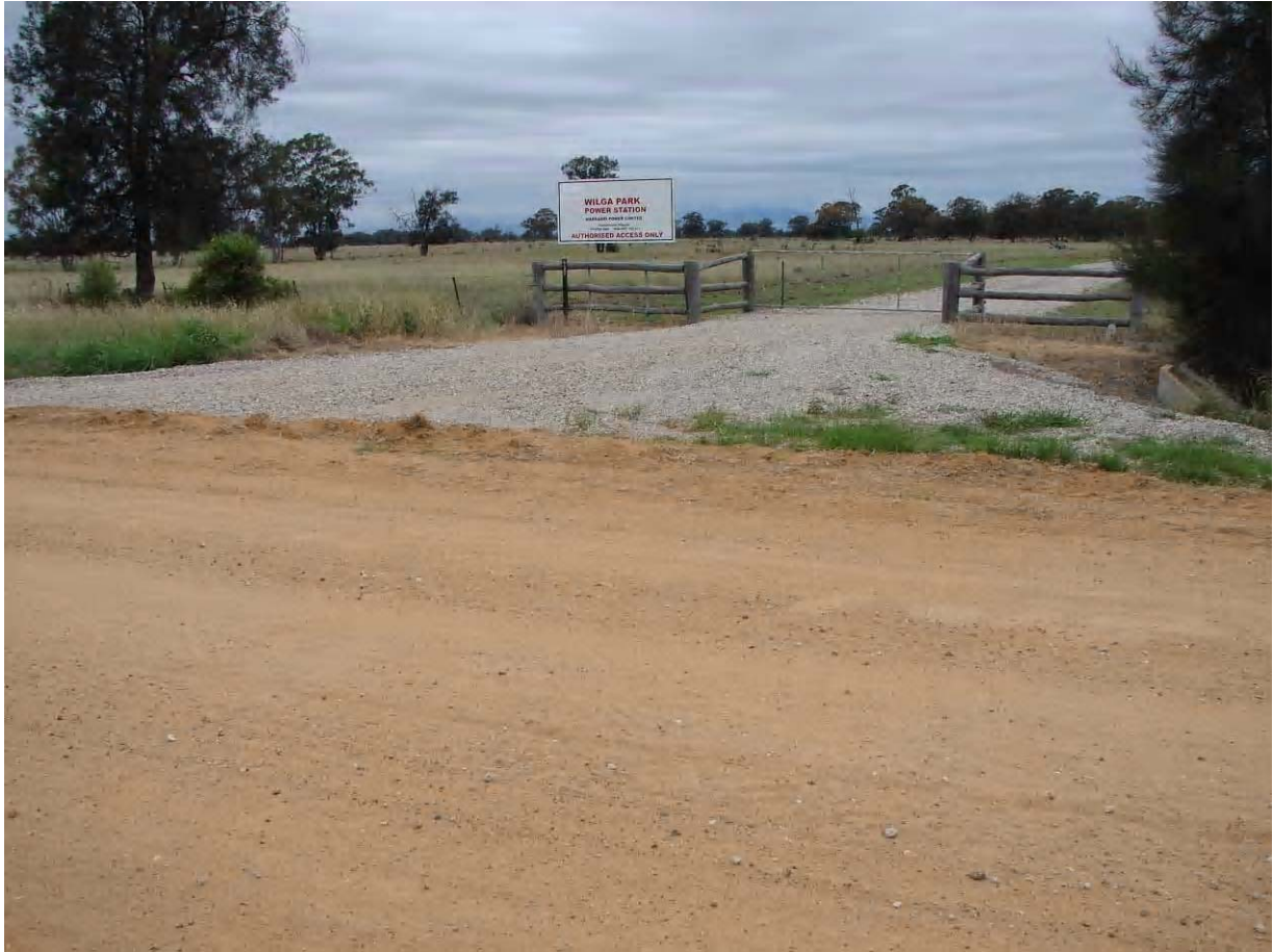
Photo 16 Entrance to Wilga Park Power Station off Kiandool Lane
