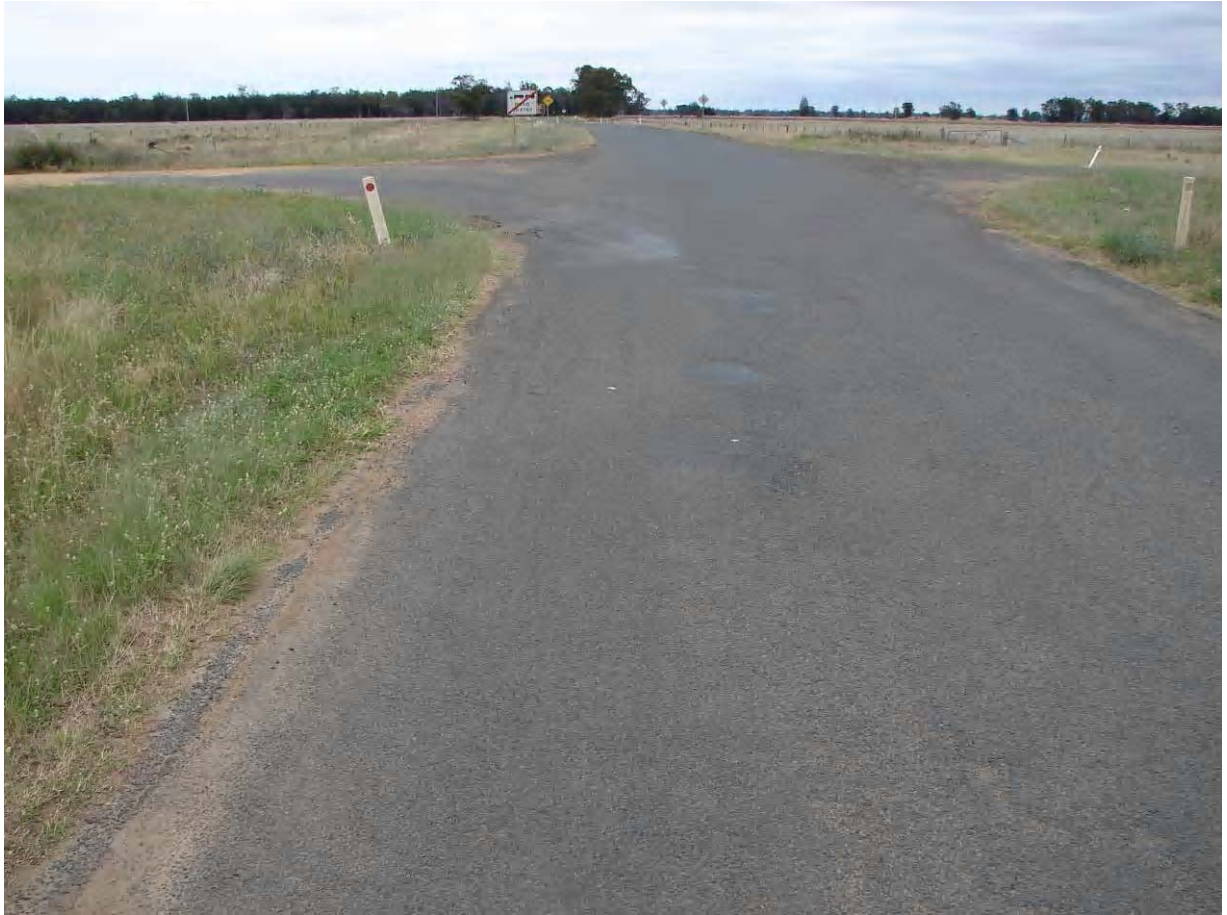
Photo 11 Kiandool Lane Intersection Facing West
