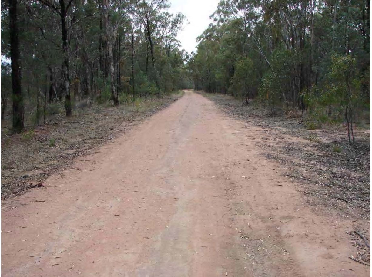
Photo 52 Dog Fence Road Facing South at Pipeline Crossing
