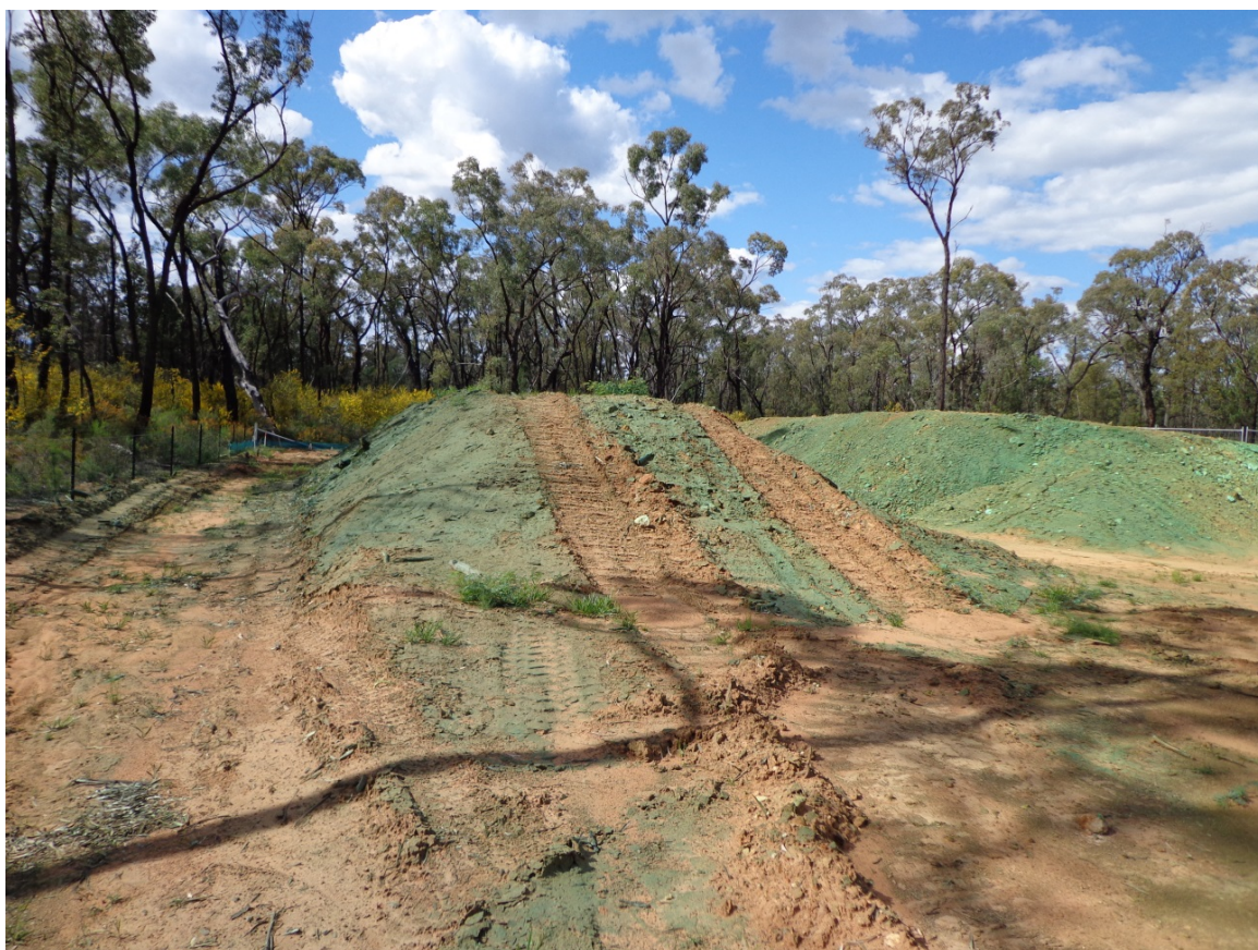
Dewhurst 31 topsoil stockpile showing disturbed polymer seal
