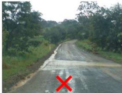
UNCONTROLLED DRAINAGE. WATER SPILLS ACROSS TRACK AT LOW POINTS, CAUSING EROSION
