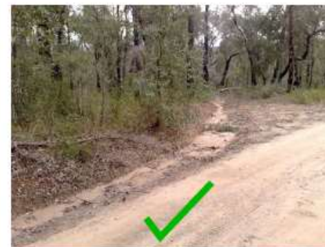
USE OF TURN-OUT (MITRE) DRAINS TO MOVE WATER AWAY FROM TRACK
