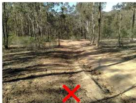
WHEEL RUTS FUNNEL WATER ALONG TRACK, CAUSING EROSION
