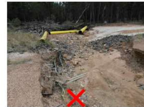
POOR STABILISATION OF WATERCOURSE CROSSINGS MEANS ADDITIONAL ONGOING COSTS FOR MAINTENANCE AND REPAIR.
