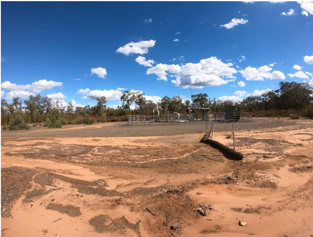
Above: Bibblewindi 24 – coir log is failing to mitigate erosion and flow of material across the site
