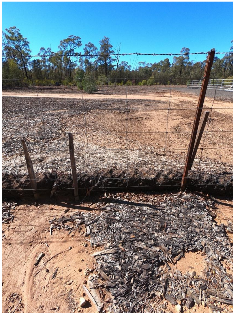
Above: Bibblewindi 12 – coir log is failing to mitigate erosion and flow of material across the site
