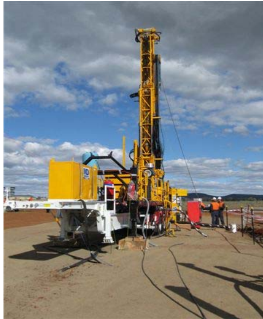
Figure 3-2: Typical Drilling Rig
