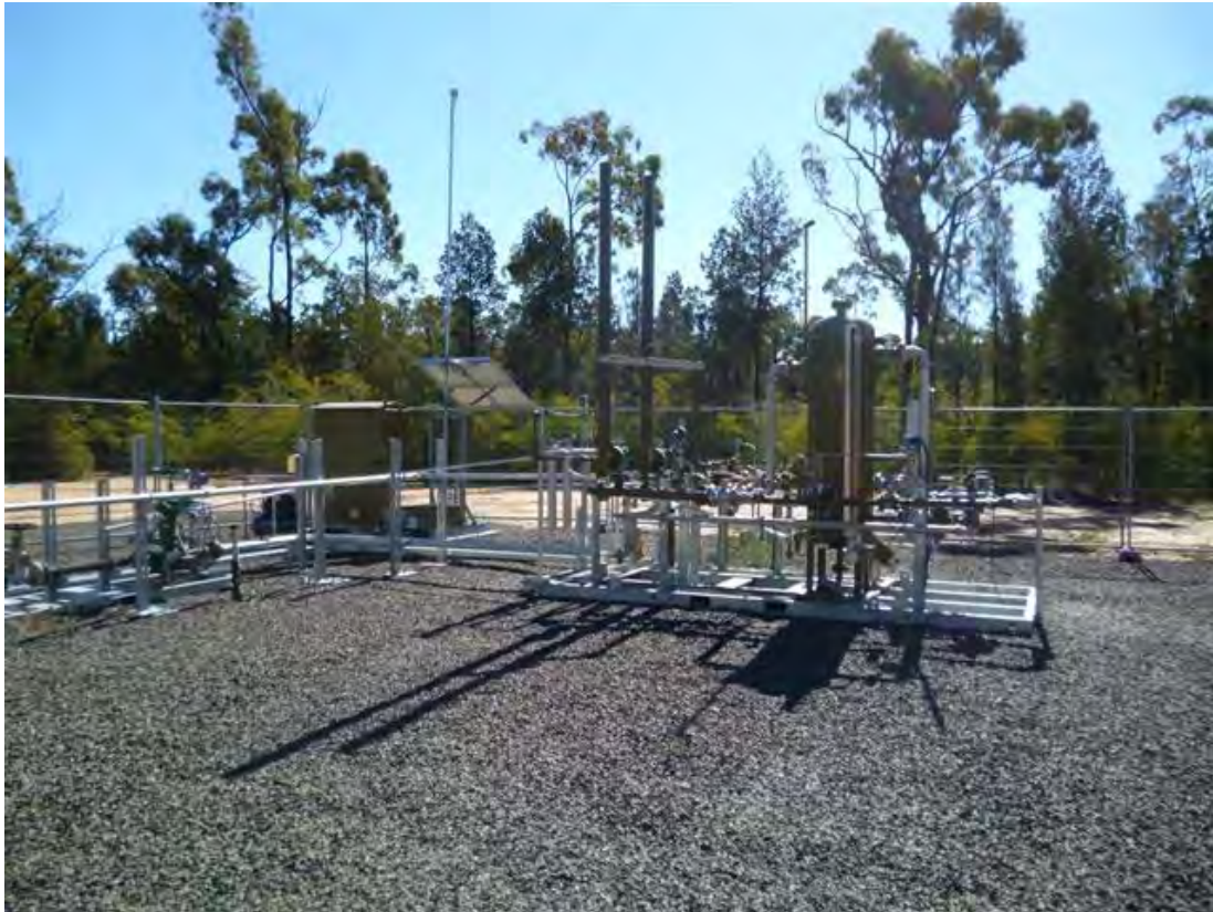
Plate 3-1 Typical wellhead separator
