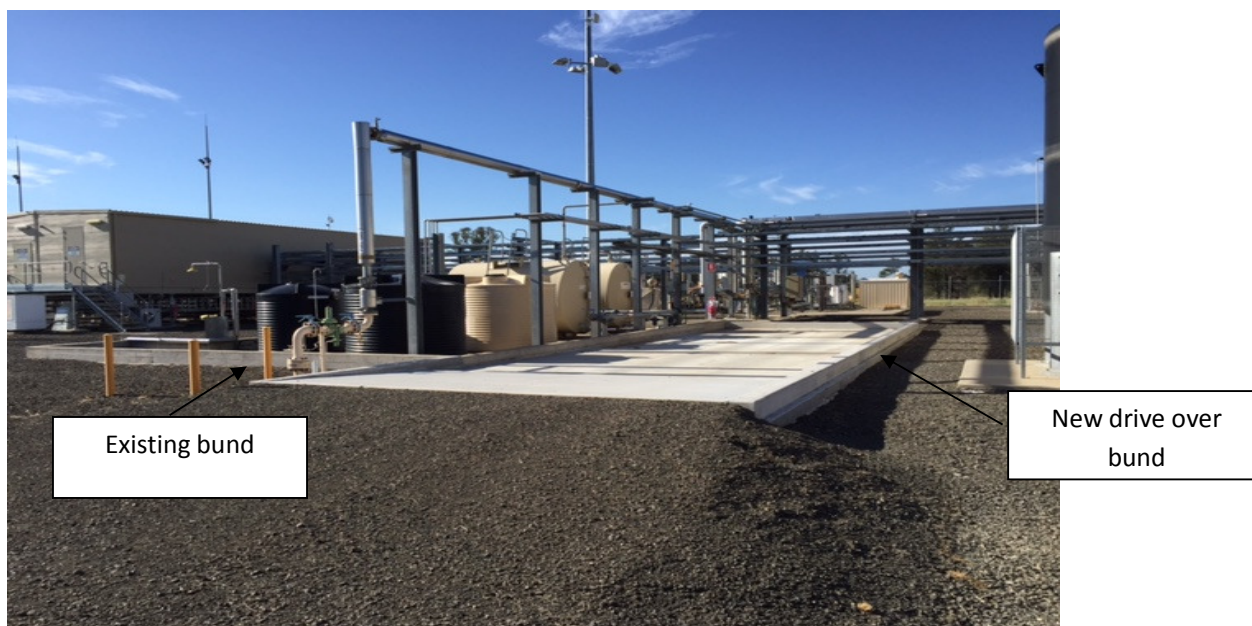
Figure 3: Wilga Park Power Station drive over bund
